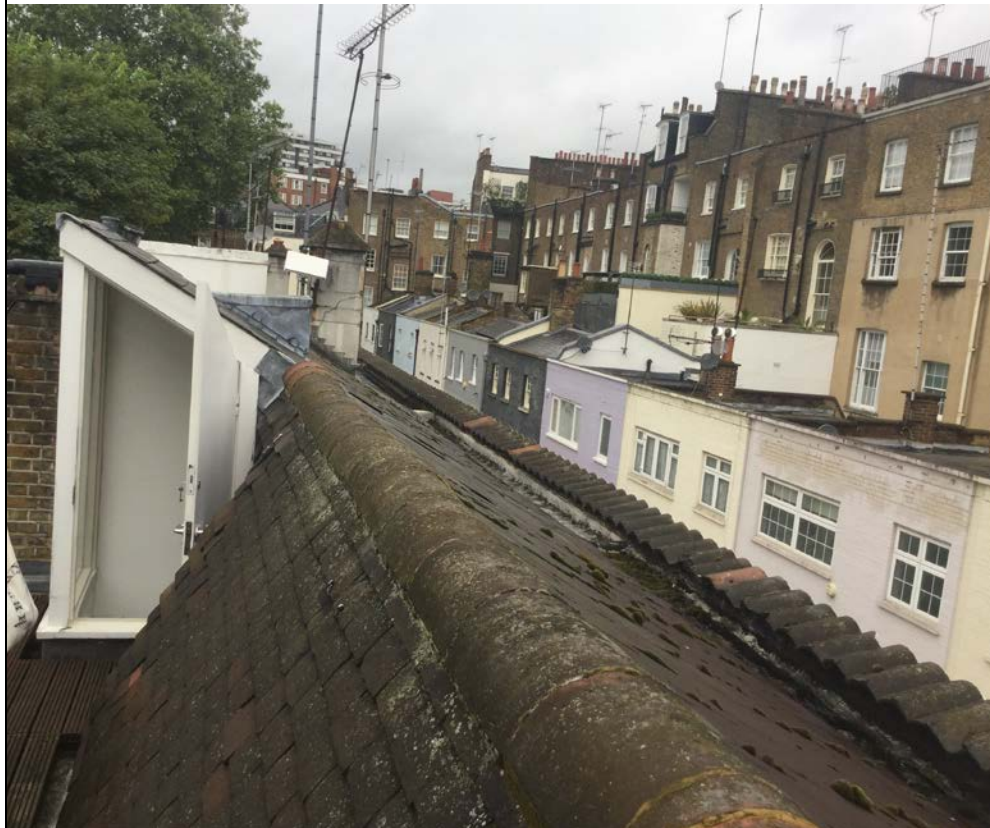
Existing Ridge line, showing relationship with the rest of the mews
