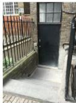
Existing steps down to rear escape stair entrance from Hallam Mews
